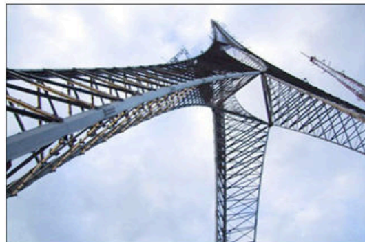
Steel structure, seen from below.
